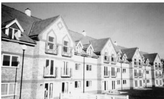
Bridgewater Court by the station, A better skyline?
