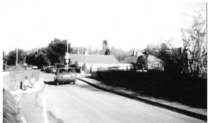
New Road Canal Bridge, Northchurch
