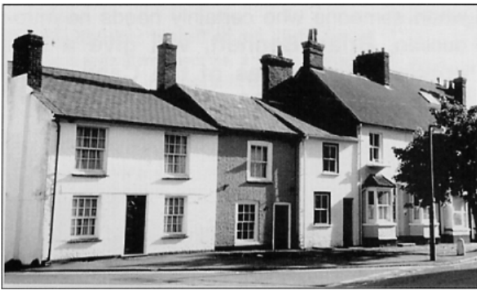
These cottages in Castle Street are in the Conservation Area, but their appearance is not fully protected by planning regulations
