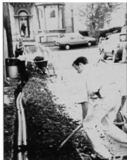
Low tech. trenches for high tech. cables in Holliday Street
