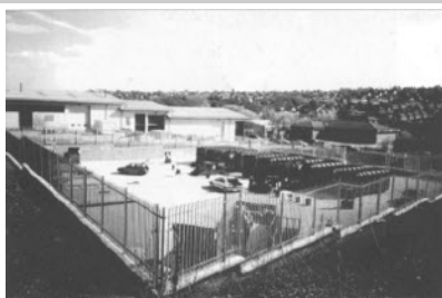
Berkhamsted's new domestic waste facility - Fully functional
