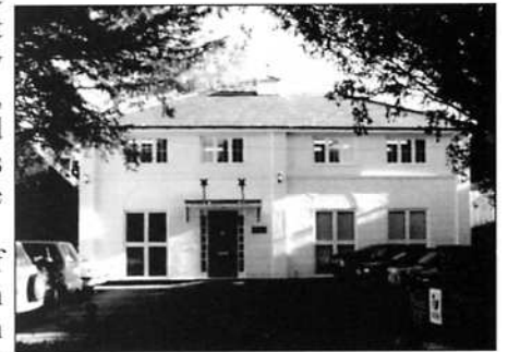
Commended in 1996. A Boxwell Road improvement
