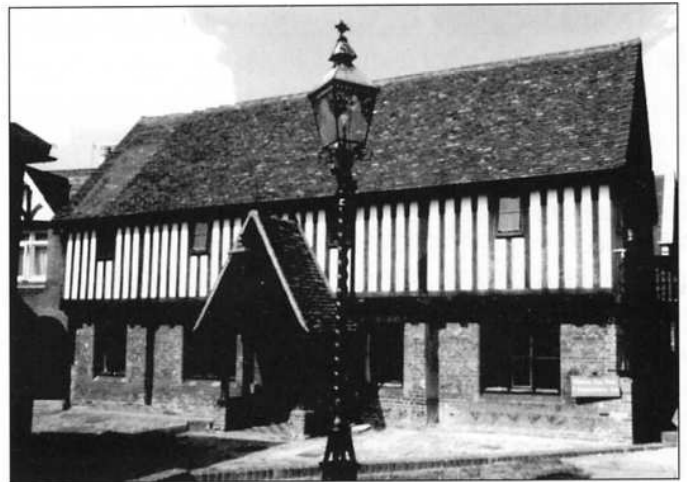
The Court House: this year's venue
