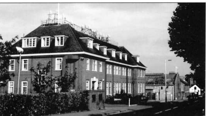
The AgrEvo site: scheduled for demolition
