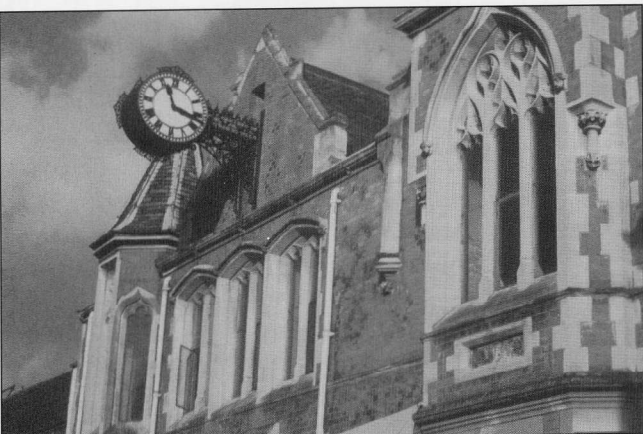
The front room of the Town Hall: to be completely restored
