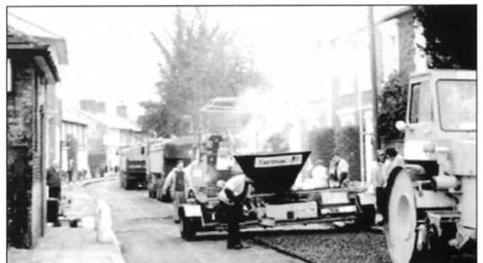
Re-surfacing Chapel Street - 1998
