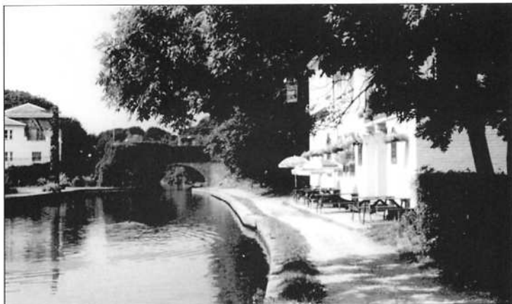
Towpath by the 'Crystal Palace': damaged
