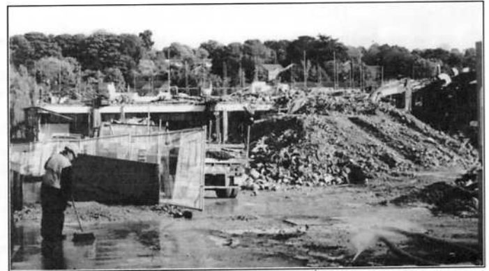
The demolition at 'Castle Quay' has opened up new vistas.
