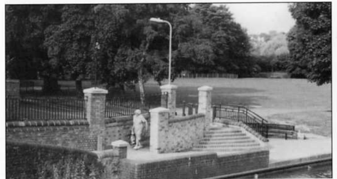
The CARP works, phase 1
