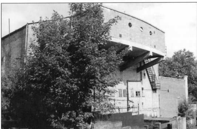
The Rex from Three Close Lane. Scope for improvement!
