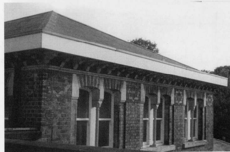
The Railway Station: not yet listed.
